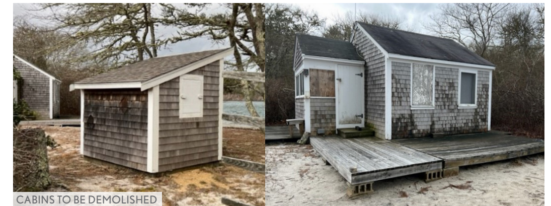
CABINS TO BE DEMOLISHED
