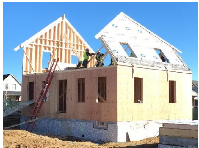
Sachem's Path, Nantucket – Under construction
