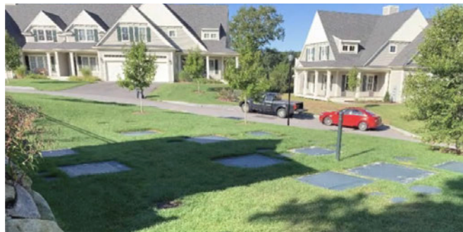
NEIGHBORHOOD WASTEWATER TREATMENT PLANT
