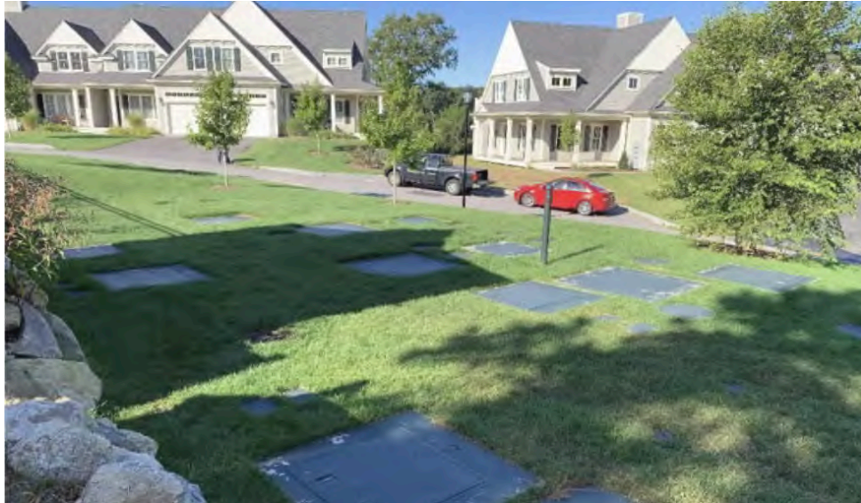
NEIGHBORHOOD WASTEWATER TREATMENT PLANT
