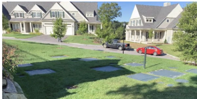
NEIGHBORHOOD WASTEWATER TREATMENT PLANT
