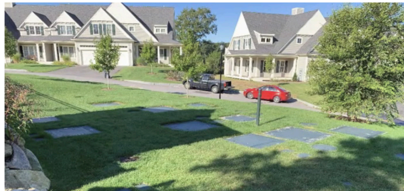
NEIGHBORHOOD WASTEWATER TREATMENT PLANT
