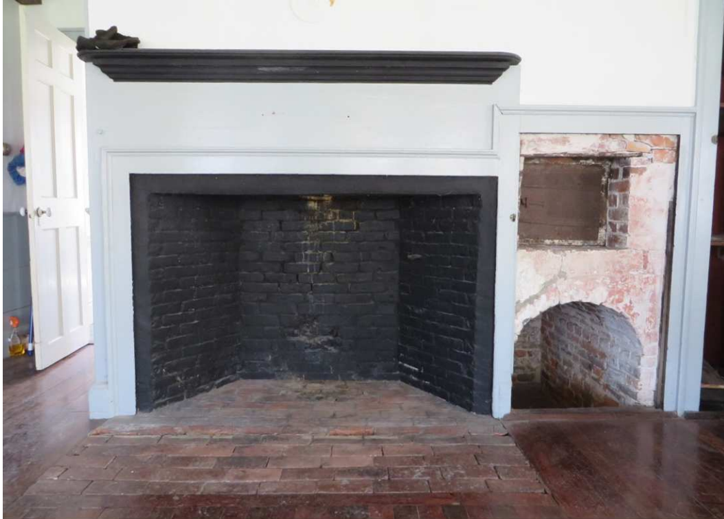
Exhibit F, Photo 51 - Cobb House interior, Kitchen Fireplace, looking south.
