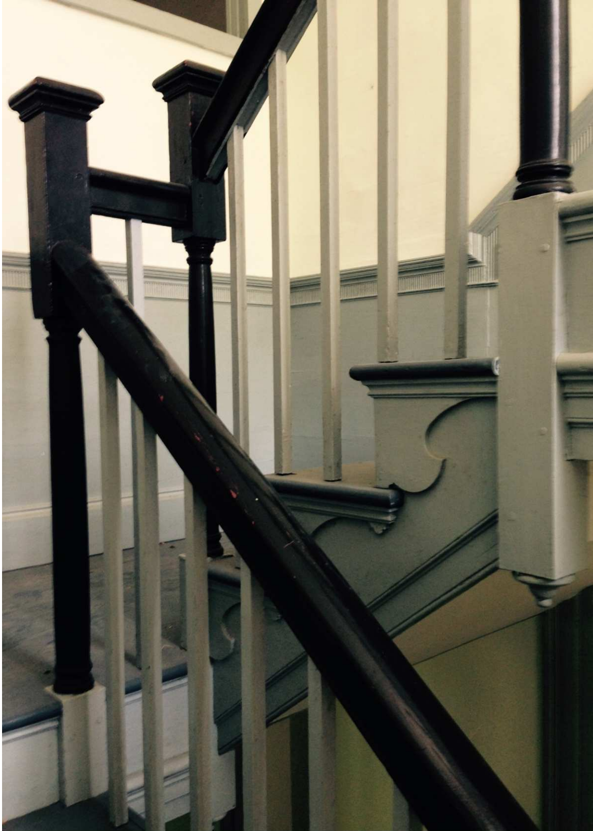
Exhibit F, Photo 50 - Cobb House interior, detail of stair, looking northeast.
