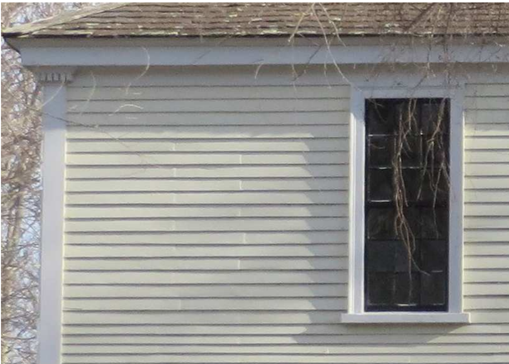
Exhibit F, Photo 10 - Cobb House, rear elevation, detail of second story window and cornerboard.
