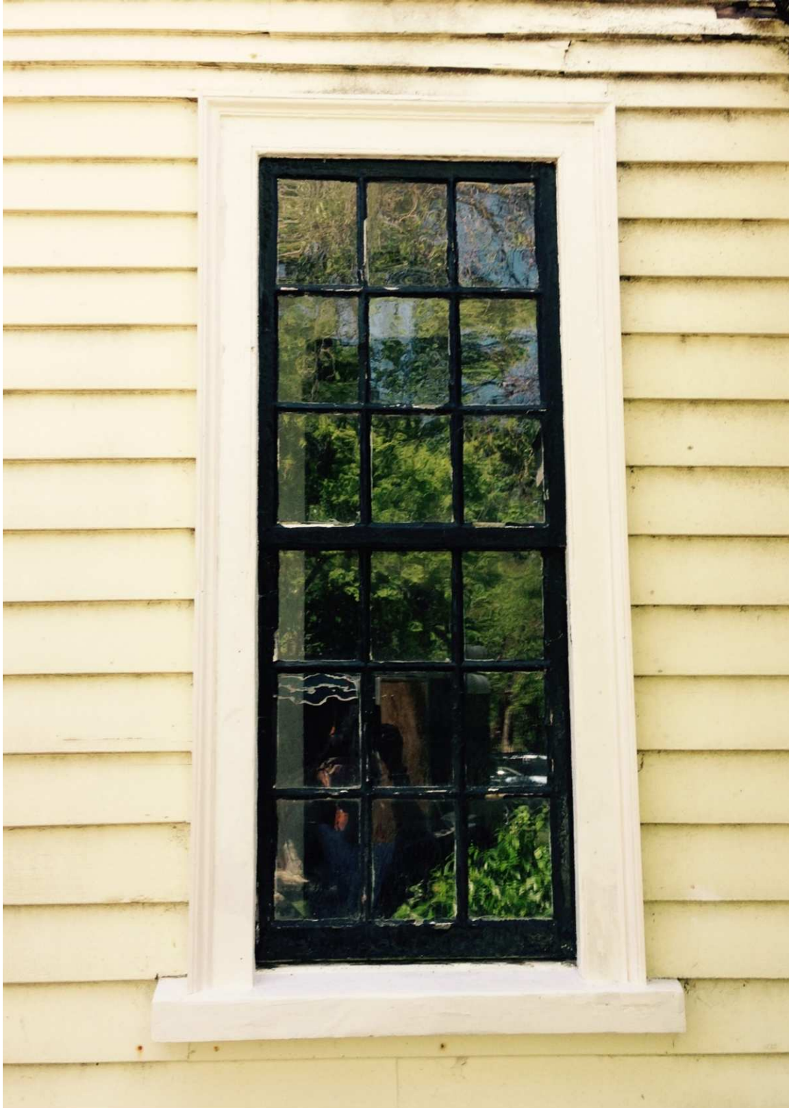
Exhibit F, Photo 11 - Cobb House, rear elevation, off-center first story window.
