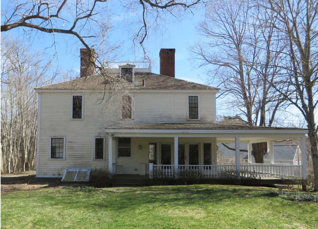
Exhibit F, Photo 9 - Cobb House, rear elevation.
