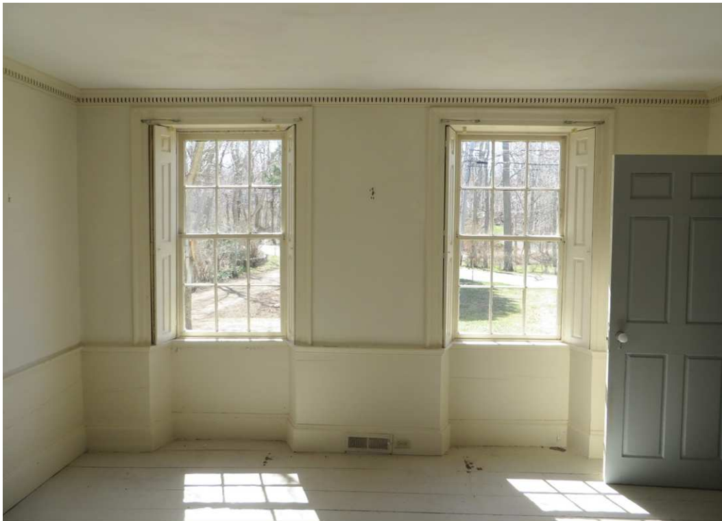
Exhibit F, Photo 21 - Cobb House interior, Southeast Parlor, looking south.
