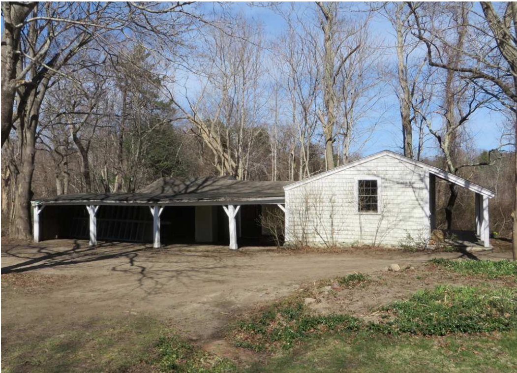
Exhibit F, Photo 54 - Cobb House outbuilding, looking east.
