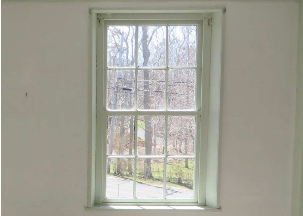
Exhibit F, Photo 43 - Cobb House interior, Southeast Bedroom, detail of window.
