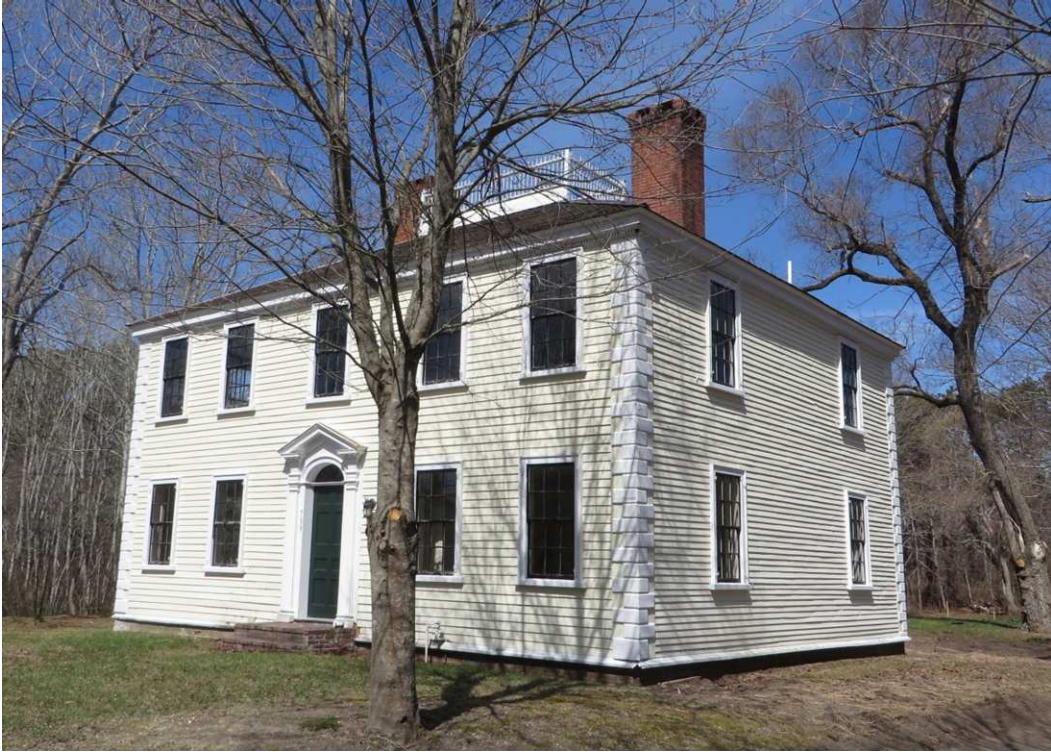
Exhibit F, Photo 2 - Cobb House, view looking northwest.
