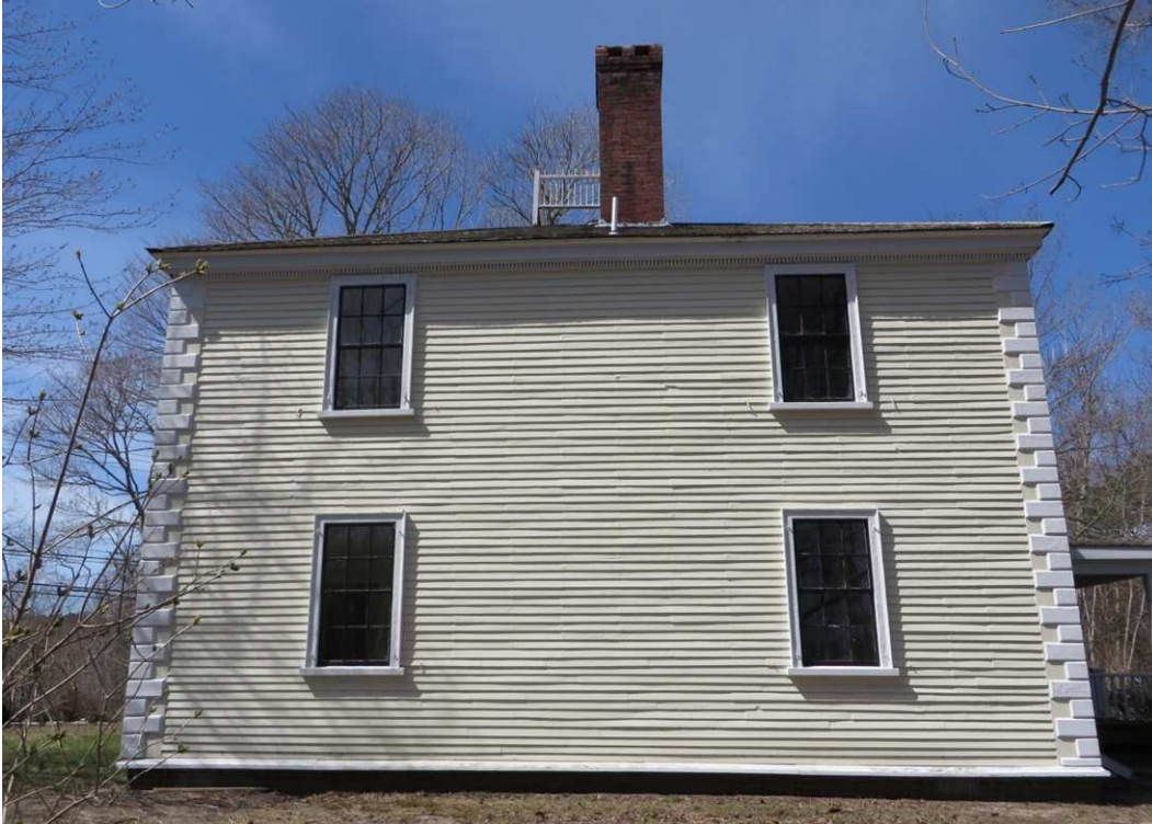
Exhibit F, Photo 7 - Cobb House, east elevation.
