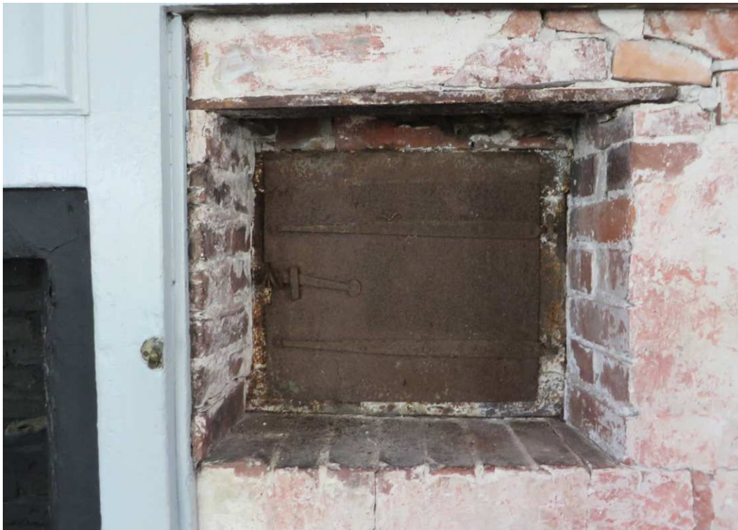
Exhibit F, Photo 52 - Cobb House interior, Kitchen Fireplace, detail of bake door.
