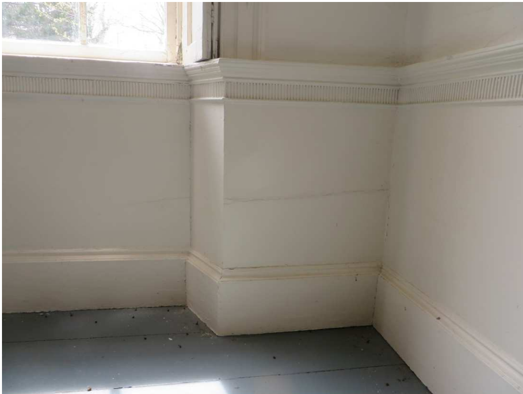
Exhibit F, Photo 17 - Cobb House interior, Southwest Parlor, detail of wainscoting.
