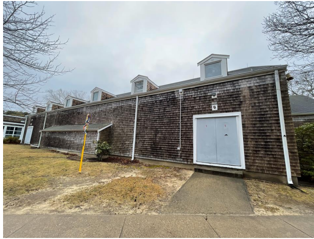
8. More examples of eroded soil and gym exit doors are not MAAB accessible.
