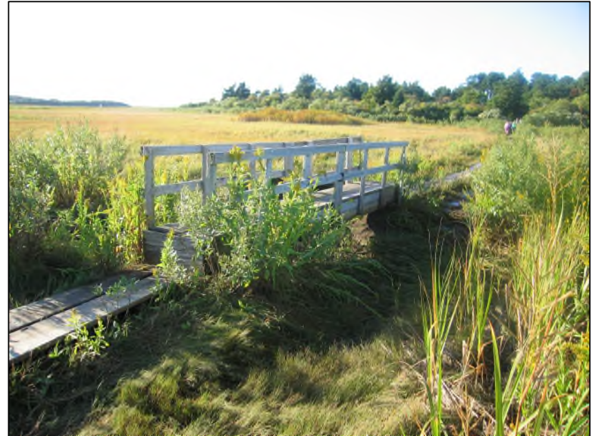
Wing Island Marsh Bridge (2008)
