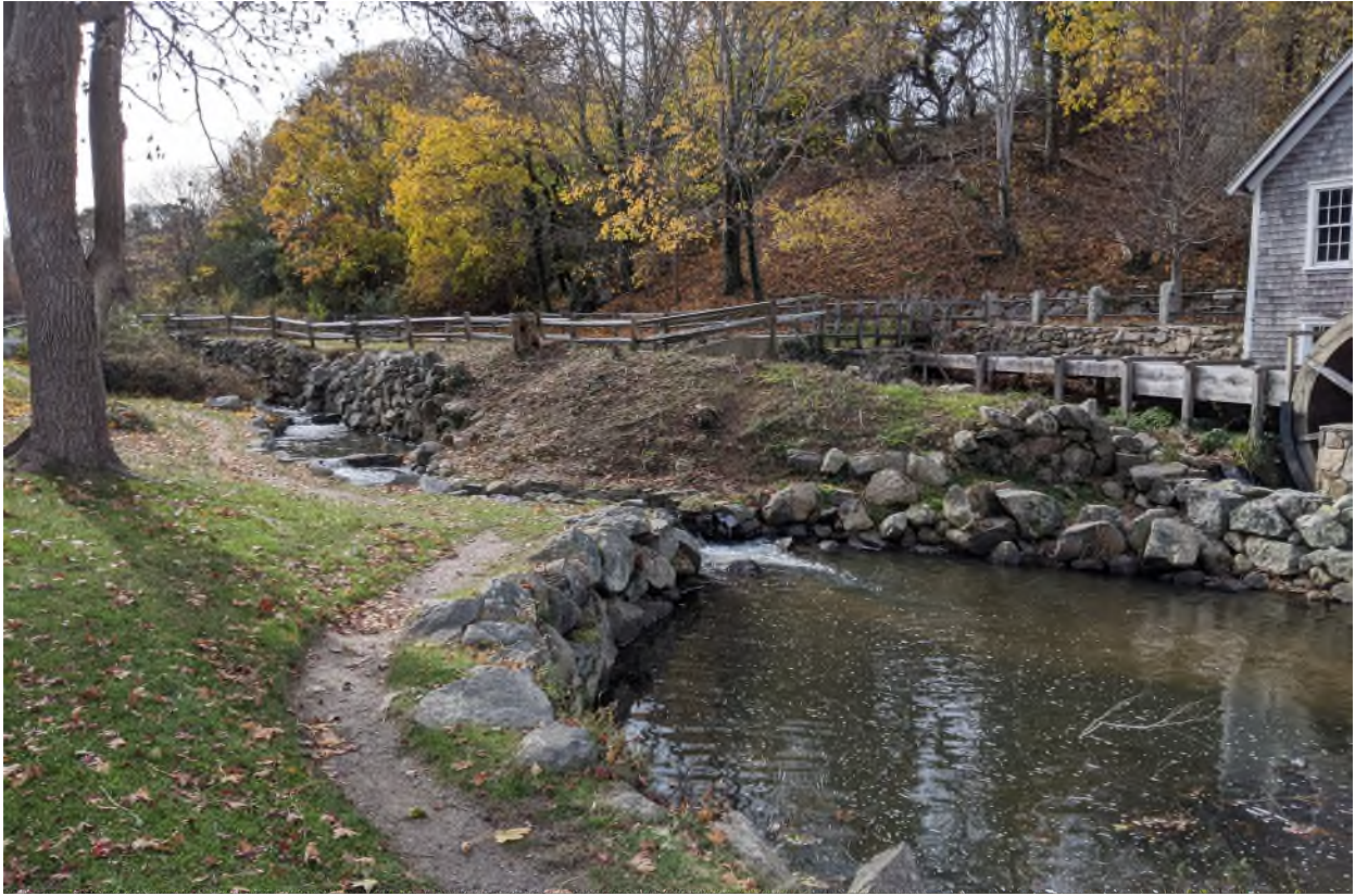
Photo 1. Retaining wall extends from near wheel south along stream to first wooden bridge.
