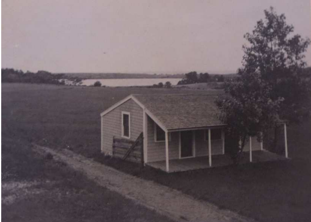
Exhibit G, Photo 5 - Outbuilding, The Den, ca. 1901.
