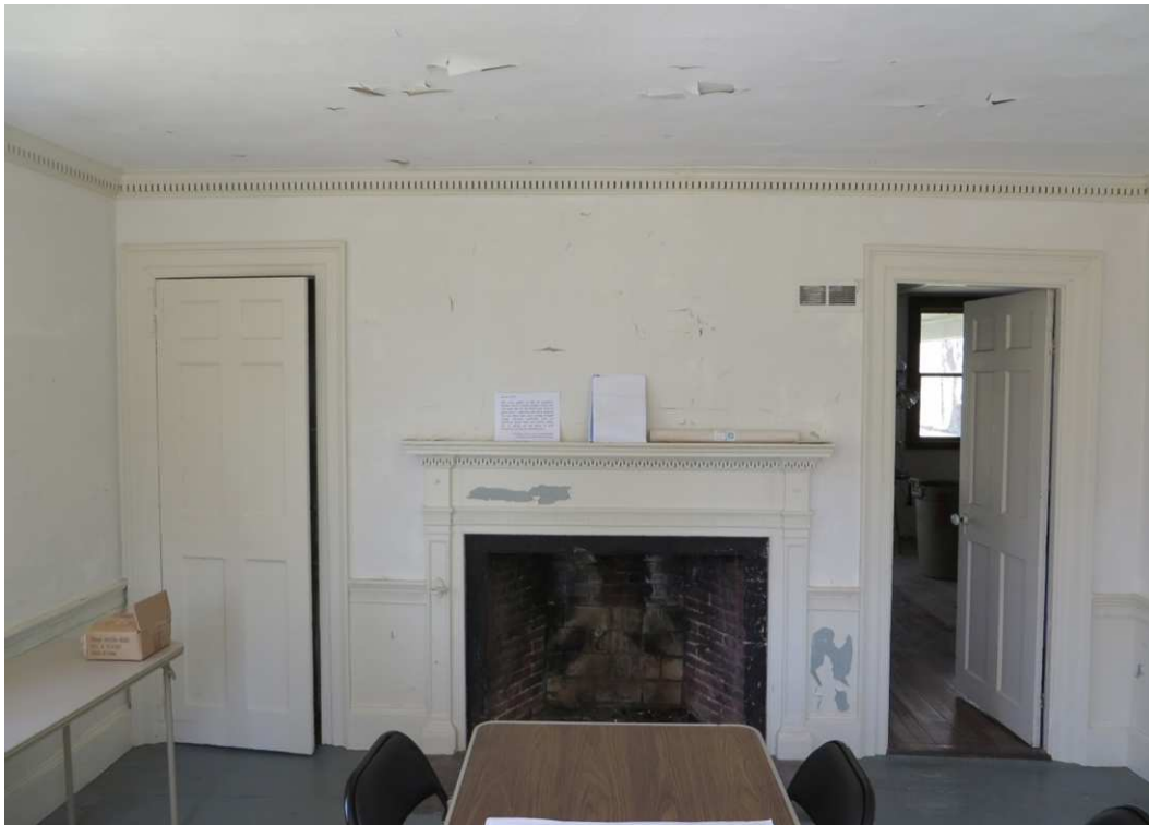
Exhibit F, Photo 15 - Cobb House interior, Southwest Parlor, looking north.
