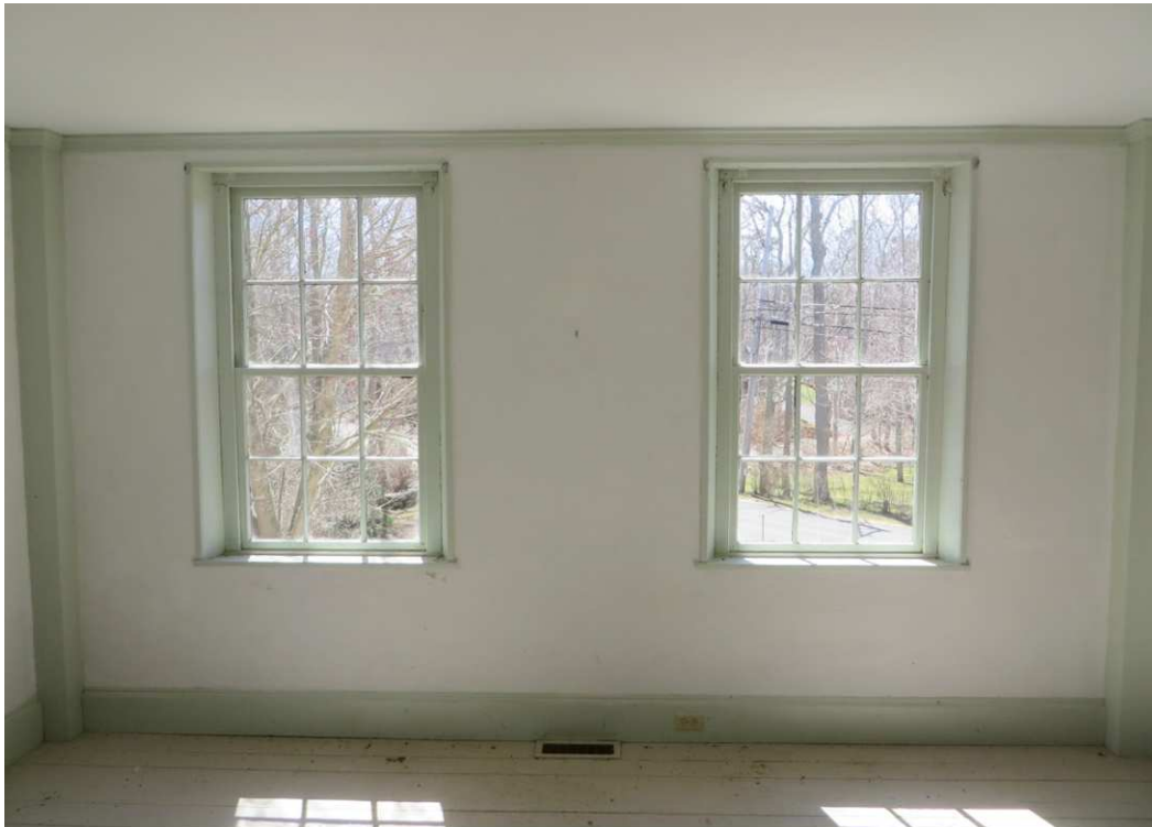
Exhibit F, Photo 38 - Cobb House interior, Southeast Bedroom, looking south.
