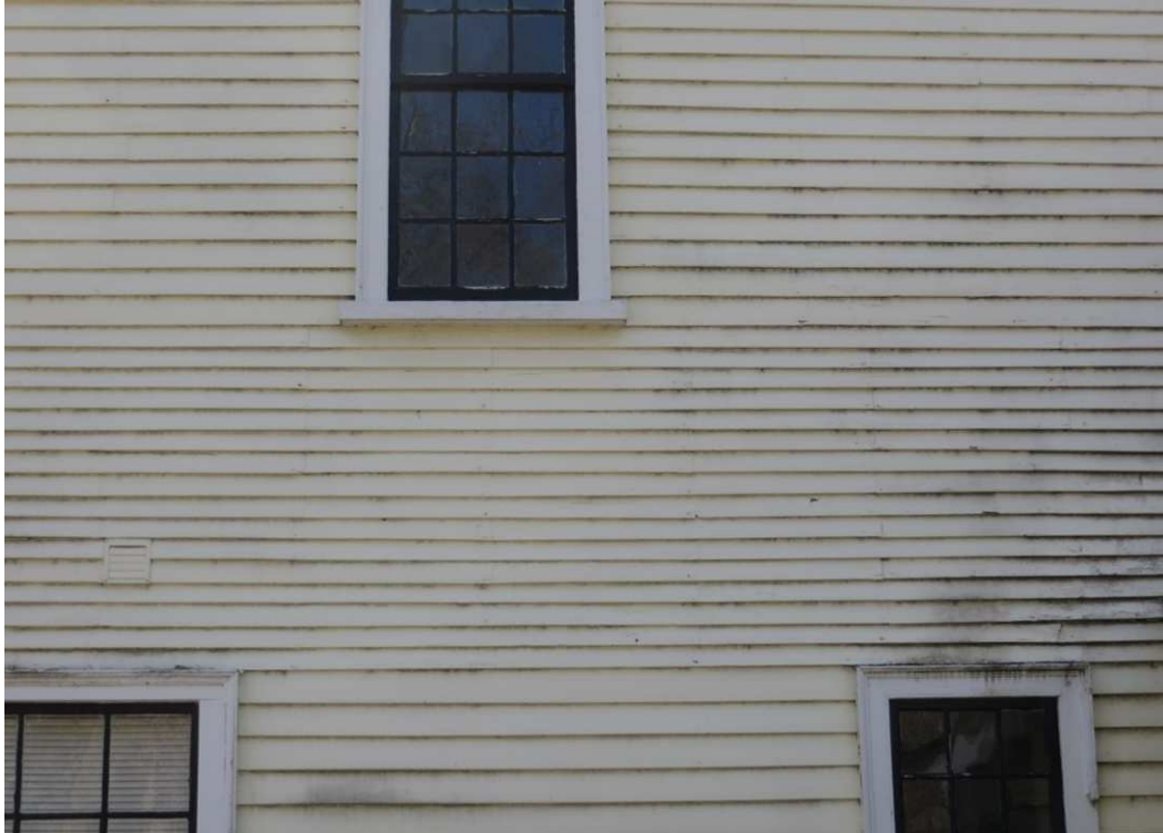
Exhibit F, Photo 12 - Cobb House, rear elevation, detail of varying-width clapboard.
