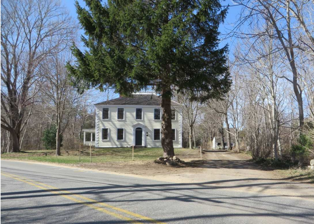
Exhibit F, Photo 1 - Cobb House, view of property, looking north.
