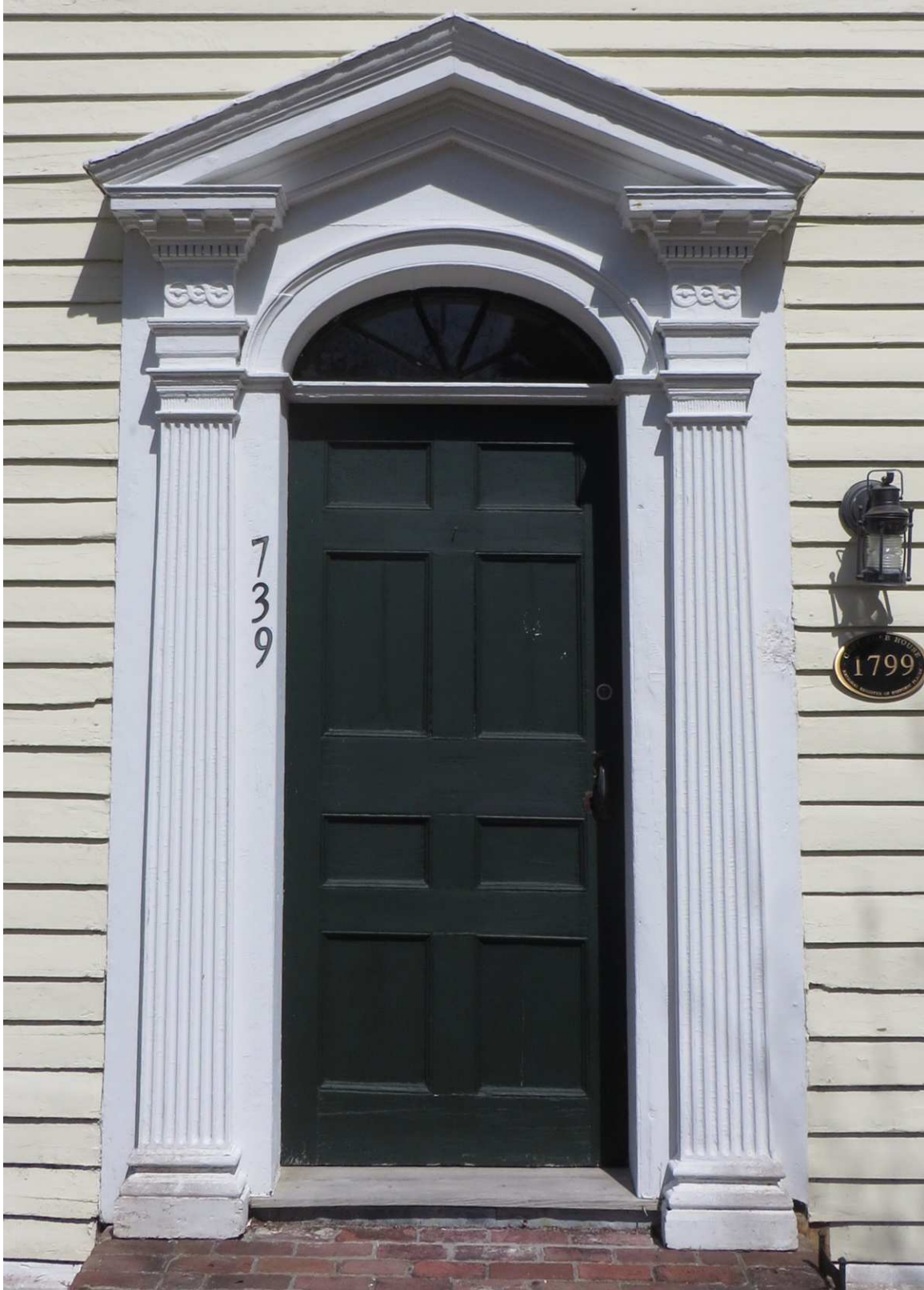
Exhibit F, Photo 5 - Cobb House, detail of front door.
