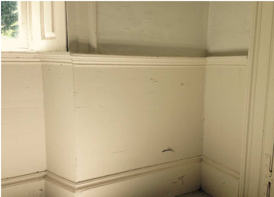
Exhibit F, Photo 25 - Cobb House interior, Southeast Parlor, detail of wainscoting, southwest corner.
