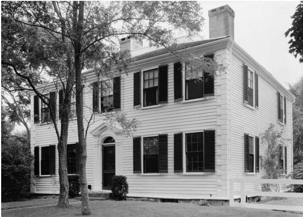
Exhibit G, Photo 6 - Cobb House, HABS, 1959.
