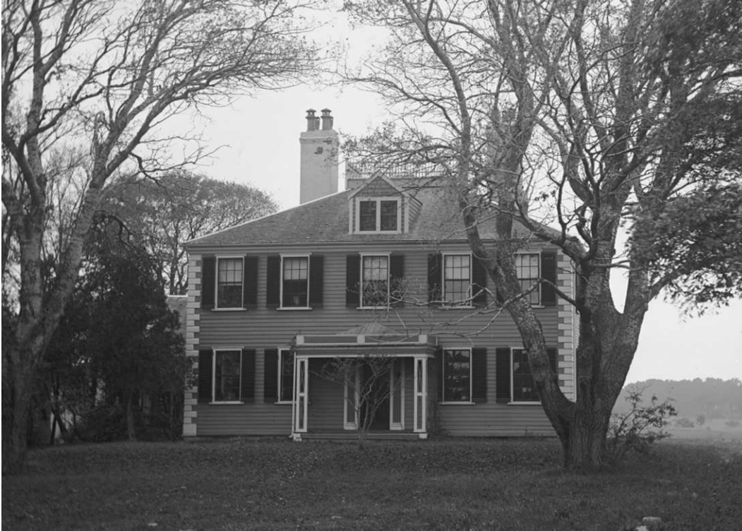
Exhibit G, Photo 1 - Cobb House, ca. 1893.
