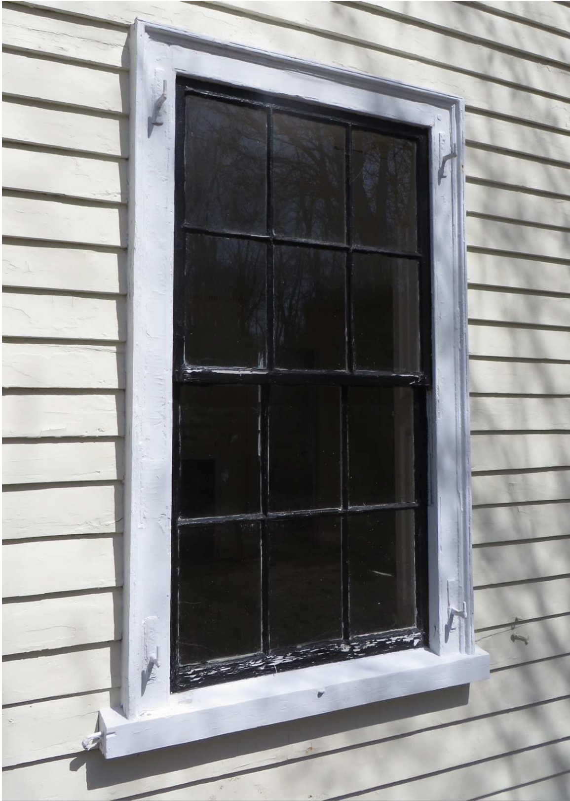
Exhibit F, Photo 6 - Cobb House, detail of window, front elevation.
