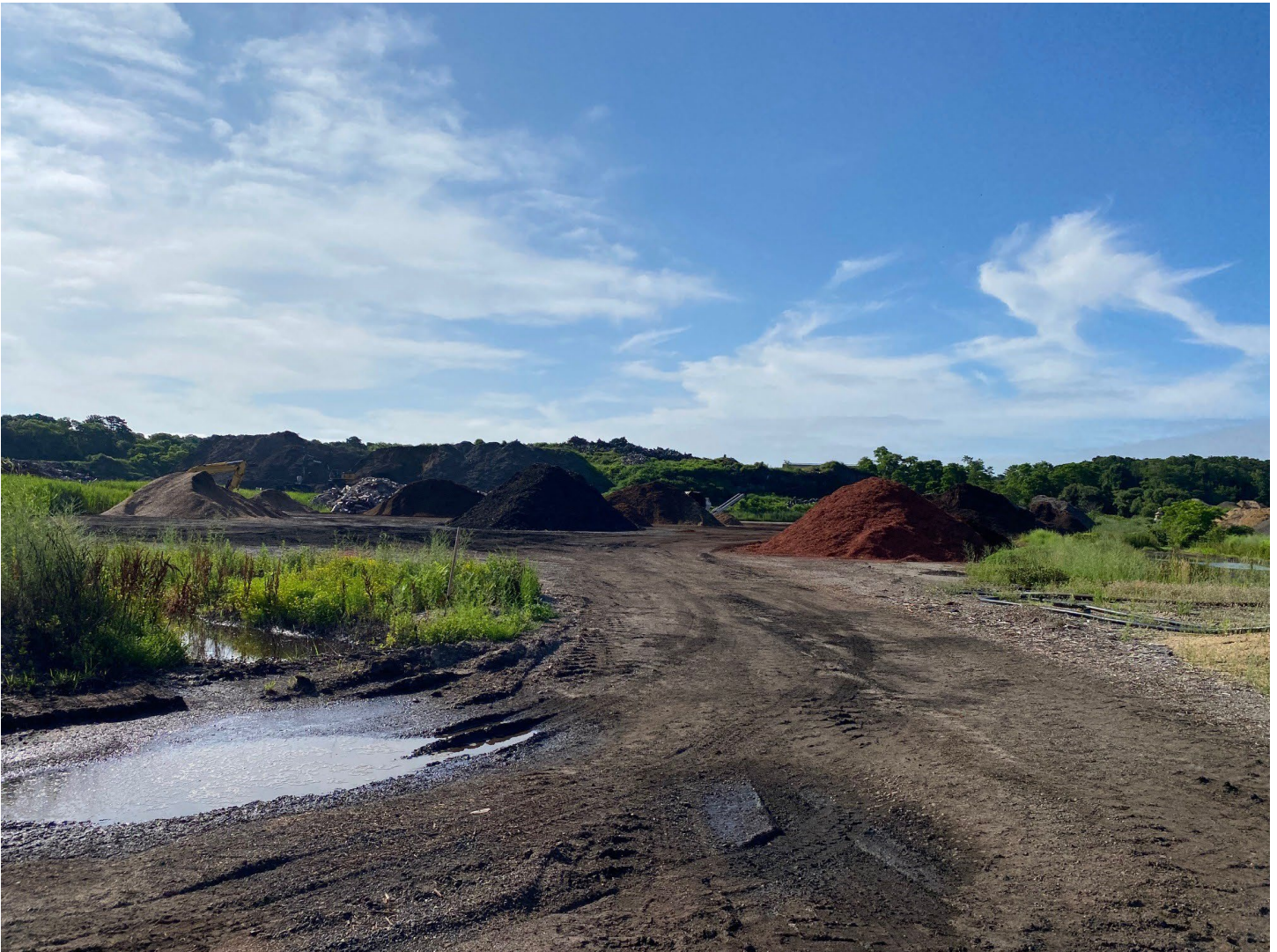
Finished landscape products and stormwater controls
