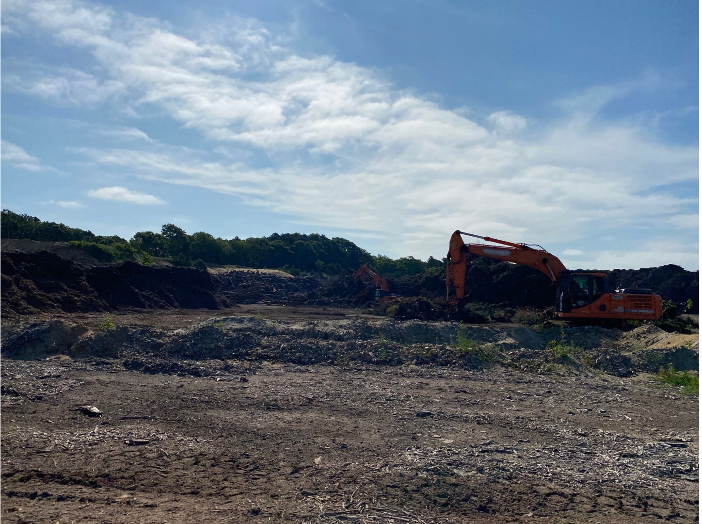
Excavators in operation
