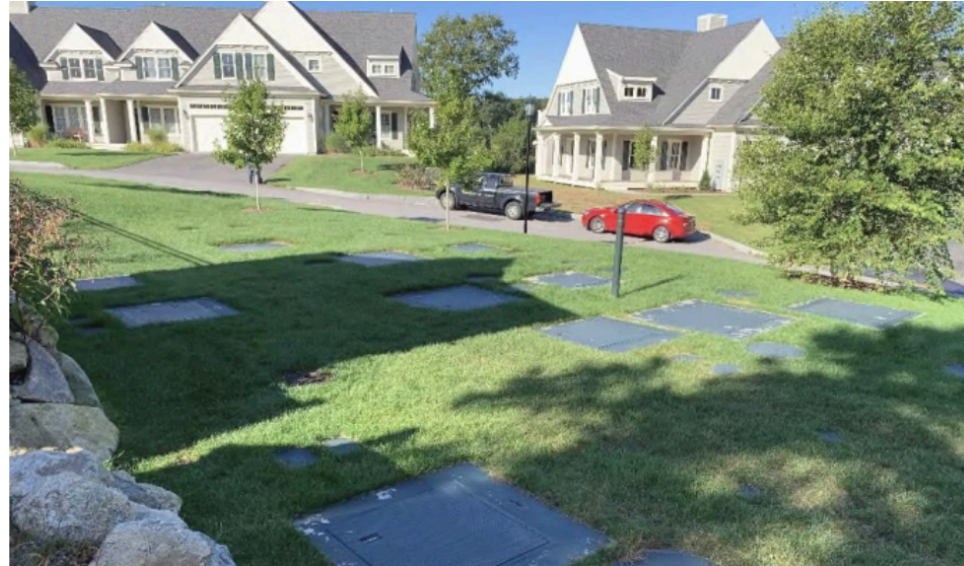
NEIGHBORHOOD WASTEWATER TREATMENT PLANT
