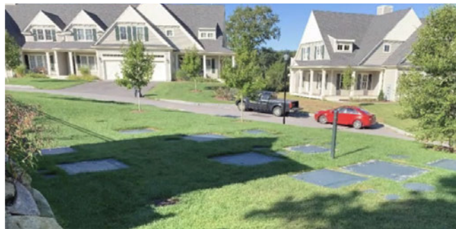
NEIGHBORHOOD WASTEWATER TREATMENT PLANT
